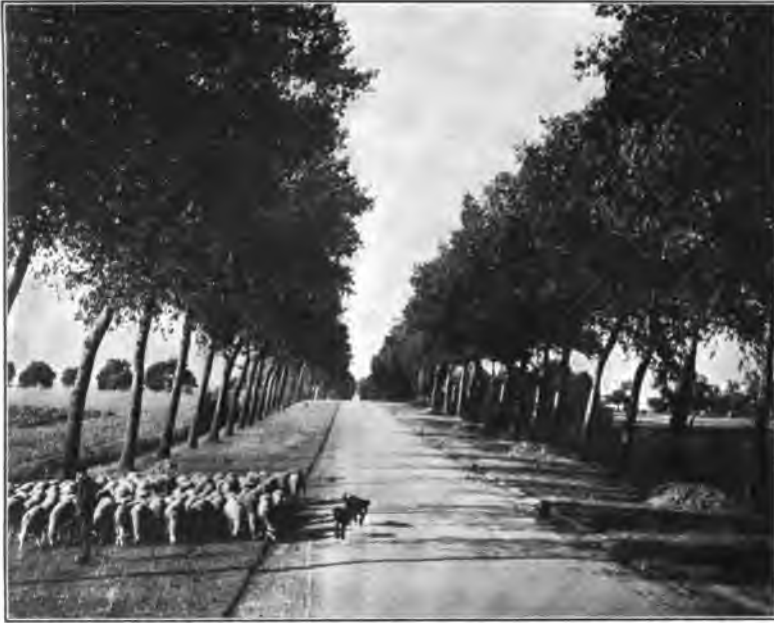
Typical road on the gently undulating plain of northern France. This is the type of surface which made possible the rapid German advance on Paris.
